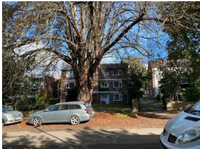
Figure 10 – Front of site
