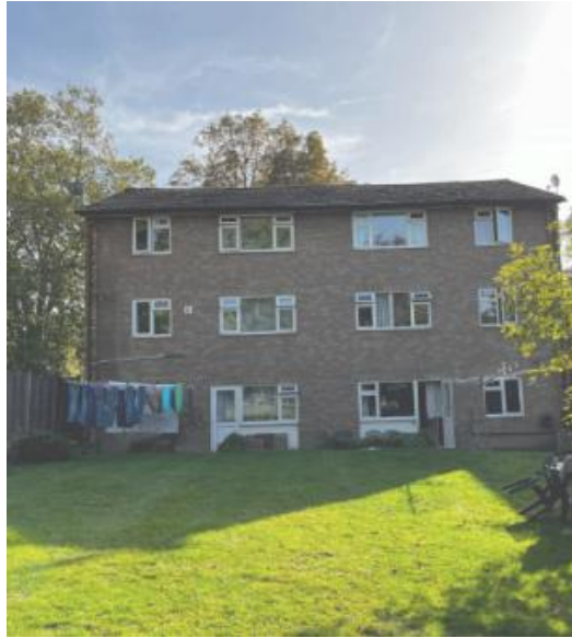
Figure 11 – rear of building
